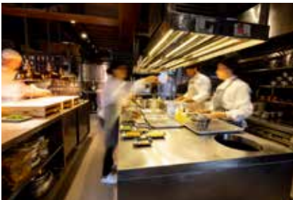
Restaurant cold rooms
