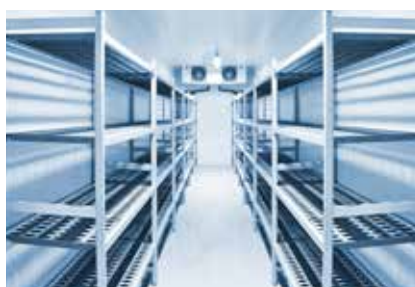
Cool room and preparation rooms
