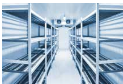
Cool room and preparation rooms
