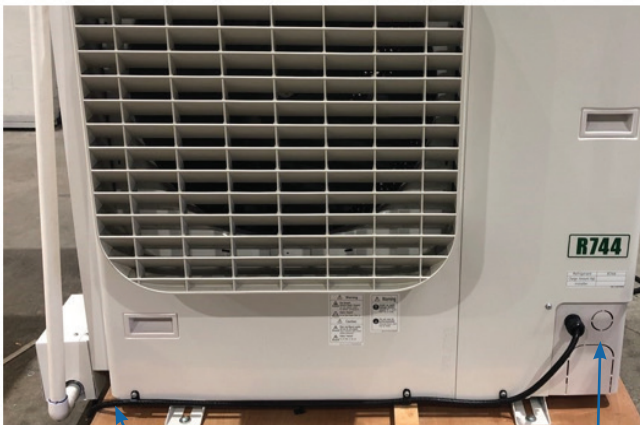
Run Cable/ Conduit toward the solenoid valve
