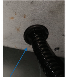
Feed cable/conduit through the Universal Bush
