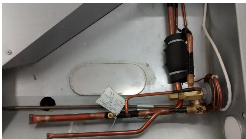
Figure 13 refrigeration access hole - base
